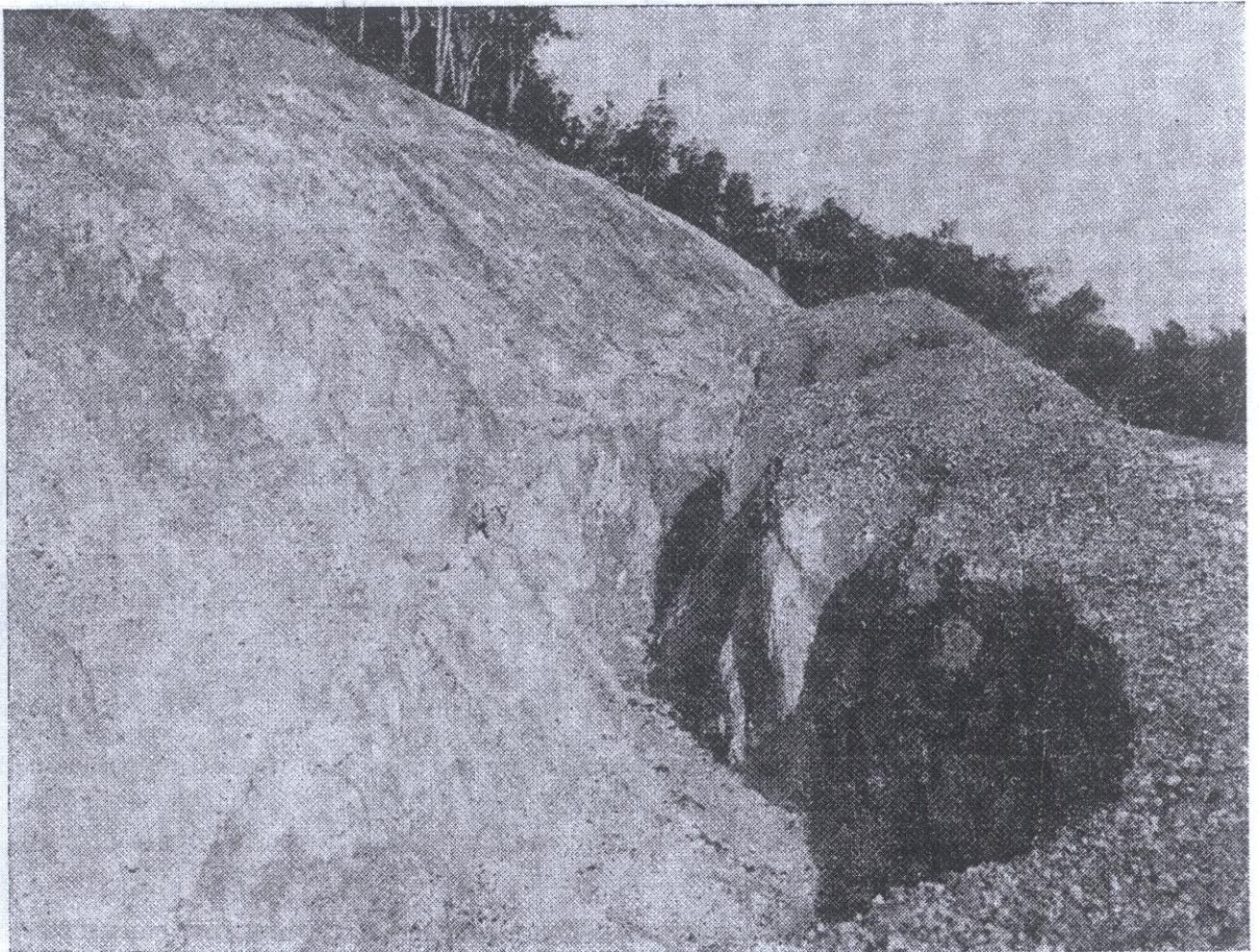
Fig. 5—Bench Erosion Developing in A New Shale Cut.
